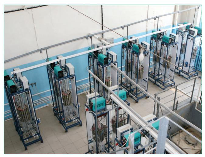
*Fig. 5.6.5.* AQUACHLOR-500 devices at the Balakovo water treatment system. In total, the system uses 76 A-500 devices, including standby ones. The daily productivity of the system in molecular chlorine equivalent is more than 900 kg.
