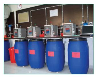
**Fig. 5.6.3.** STEL devices in a 1000-bed tuberculosis hospital in Tbilisi, 2004. Anolyte ANK produced by the devices, is fed from the storage tanks to the wastewater flow in a proportional amount, automatically controlled by a system of valves and level sensors. The devices operate in automatic mode, providing a constant maximum level of Anolyte ANK in storage tanks.
